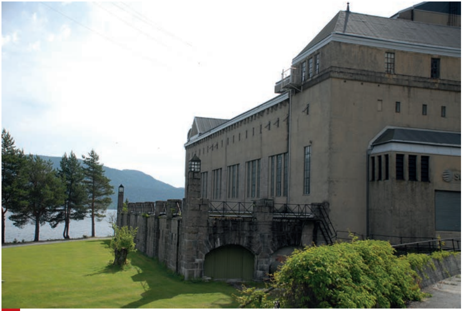
Øvre Eiker, Hakavik hydropower station. Photograph by Ulf Ingemar Gustafsson, 2014. • Øvre Eiker, vodní elektrárna Hakavik. Foto Ulf Ingemar Gustafsson, 2014.
