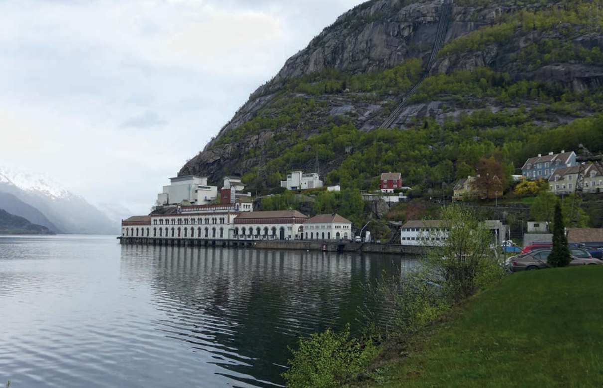
Tyssedal, hydro-electric power plant, Norwegian Museum of Hydro Power and Industry. Photograph by Michaela Ryšková, 2015. • Tyssedal, vodní elektrárna, muzeum. Foto Michaela Ryšková, 2015.
