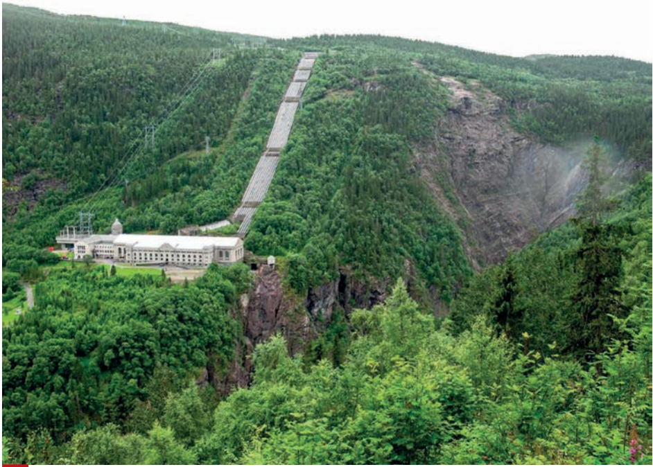
Rjukan, Vemork Power Plant by the river gorge. Photograph by Trond Taugbøl. • Rjukan, elektrárna Vemork Power Plant u říční rokle. Foto Trond Taugbøl.
